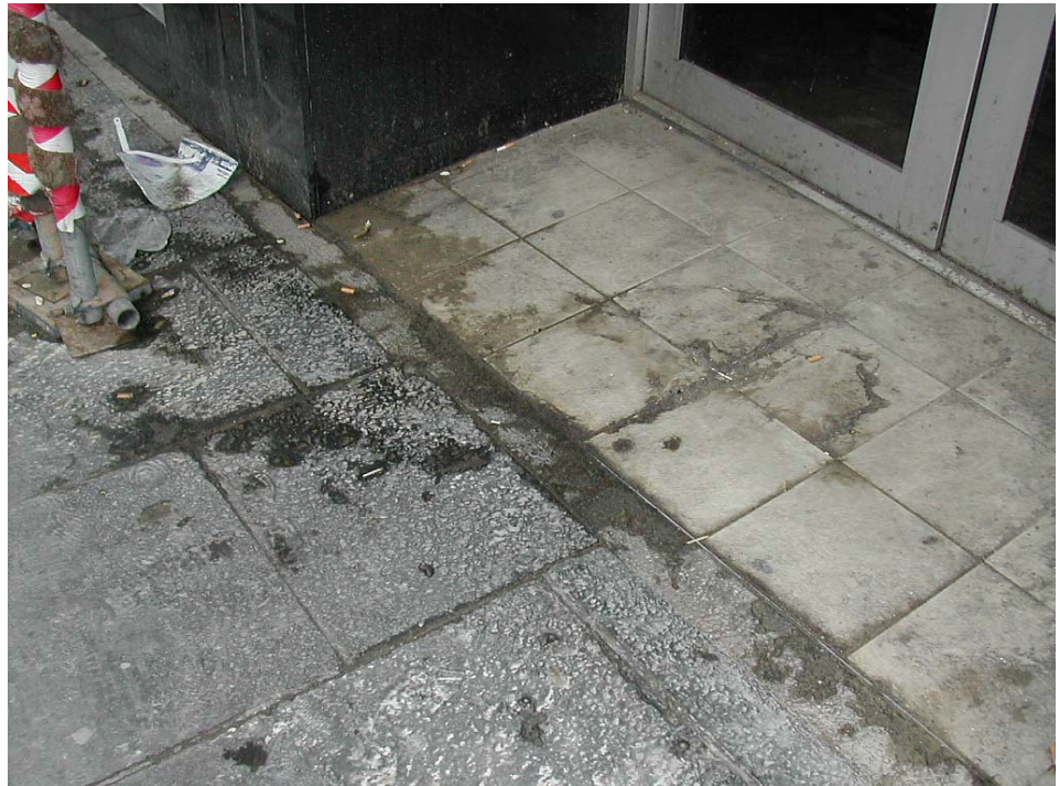
Doorways on the East side of North Bridge, near the top.
